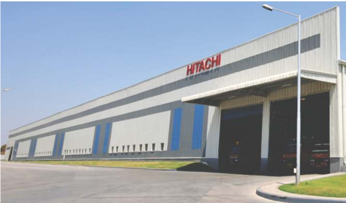
ANNA ISD | Sector: Multi-use Facility | Location: Texas, USA Area in sq m: 5,667 | Tonnage in mt: 370
